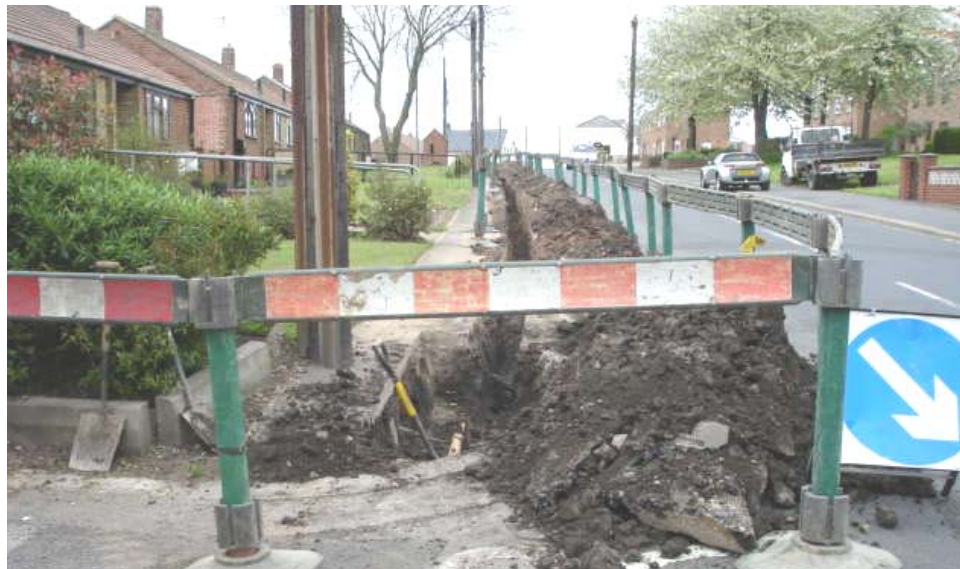
Utility works at High Pittington – No provision made for pedestrians
